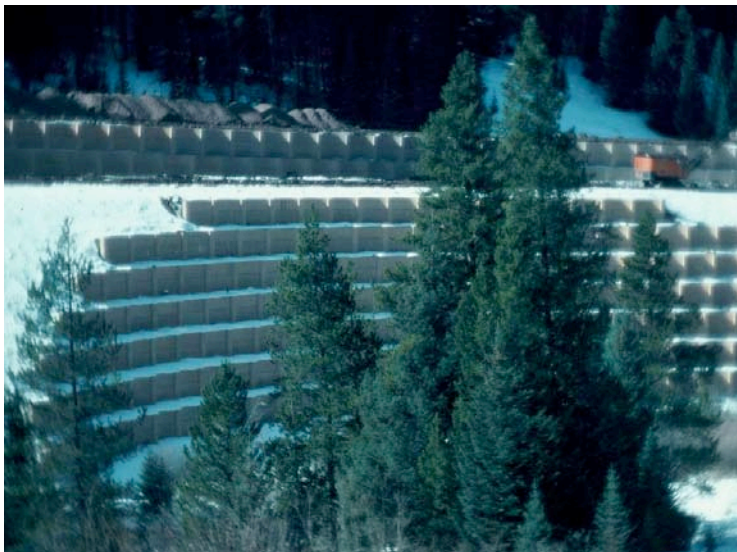
60 FOOT TALL PLANTER BOX WALL ON VAIL PASS I-70
