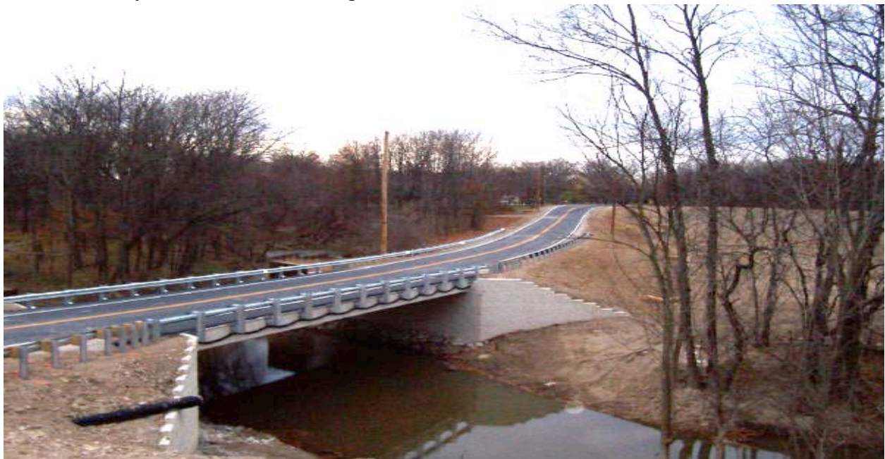
DEFIANCE COUNTY, OHIO BRIDGE ON GRS/GCS® ABUTMENTS
