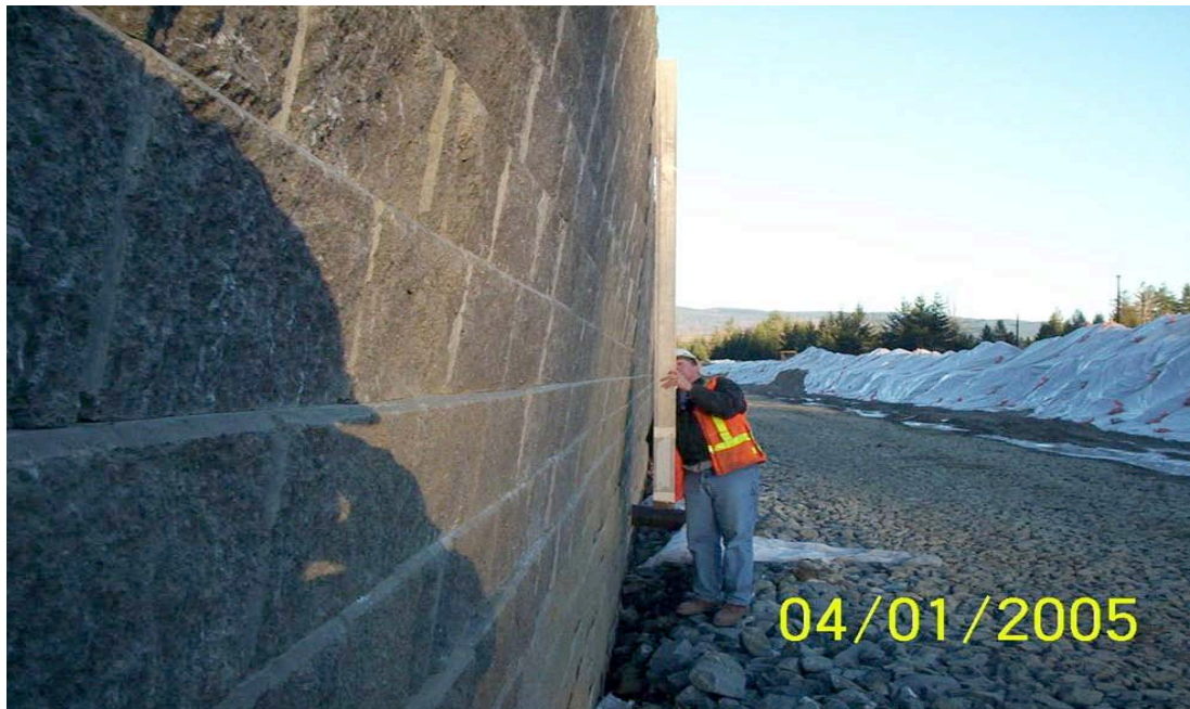
8” of negative batter along a 10’ straightedge.
